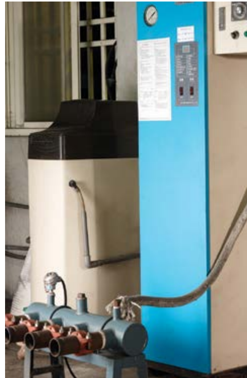
Laboratory hot water testing
